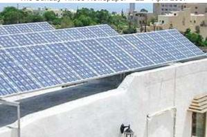
A typical solar photovoltaic grid-connected system installed in Madliena and used for generating electricity for home use. The system generates close to 10 units of electricity everyday and offsets three tonnes of carbon dioxide per annum that would otherwise have been generated at the power station for the same amount of energy.
